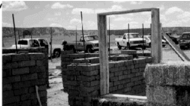
Adobe blocks were dry stacked to form the adobe walls in the demonstration house at Ganado.
