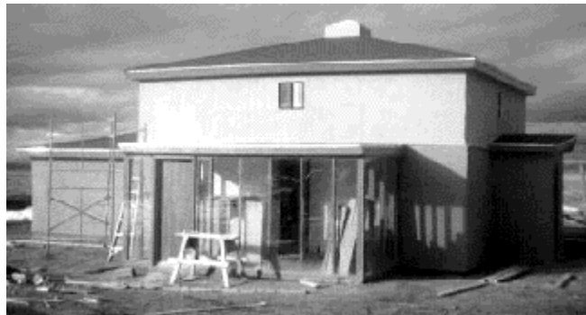
Straw-bale/adobe prototype home under construction (south-west elevation).
